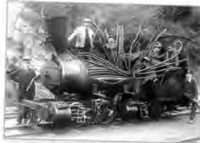
Boiler accidents were prevalent before the establishment of codes and standards.
