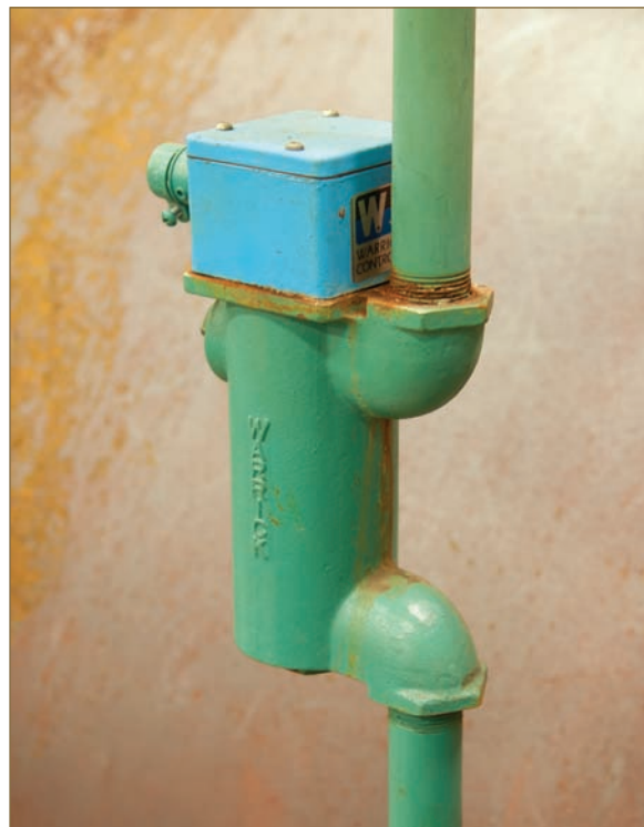
▲ Probe-type low-water cutoff
