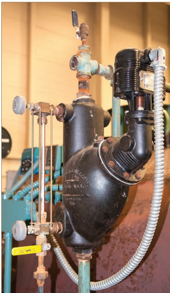
◀ Float-type low-water cutoff
