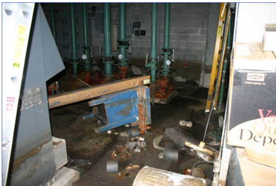
Flood damage to the mechanical room of Benjamin Franklin High School in New Orleans.
