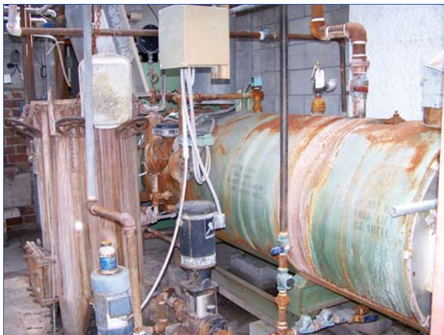
The boiler return tank/hot water preheater and boiler feed pump ruined and rusted after sitting in 6-feet-deep flood water. Equipment owned by Eric and Mary DuBuisson at Slidell Cleaners of Slidell, Louisiana.
