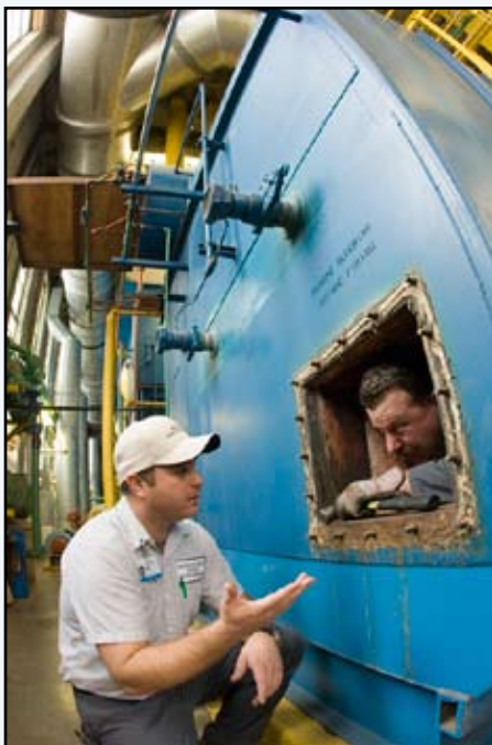
Boiler operators Tom Looker, left, and Woody Sarver work on boiler No. 6.
