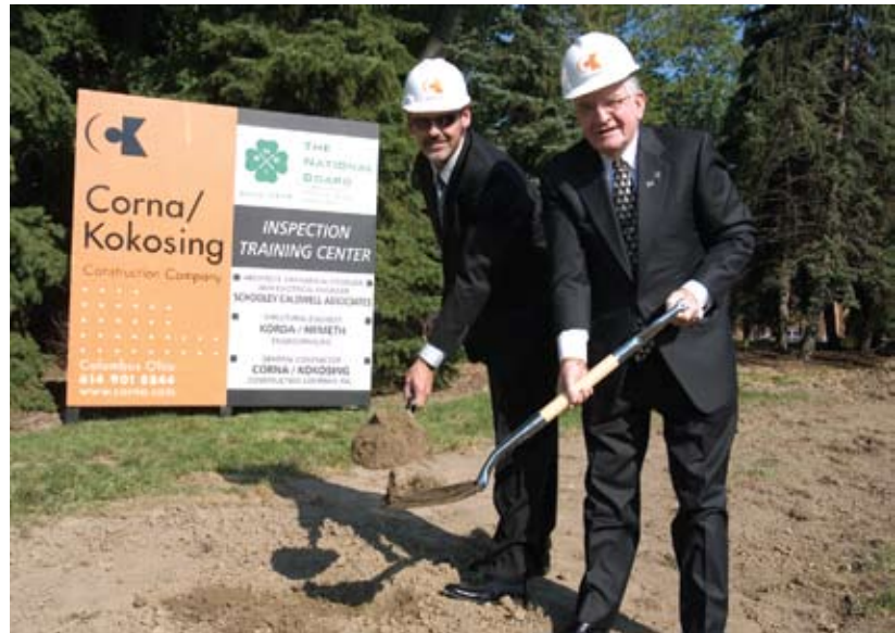
David Douin (left) and Donald Tanner perform groundbreaking duties.
