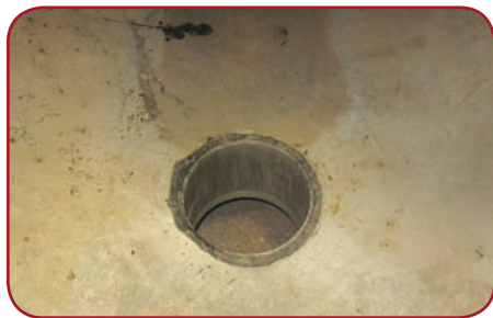
Figure 1. The inside of a pressure vessel nozzle that has been in service.
