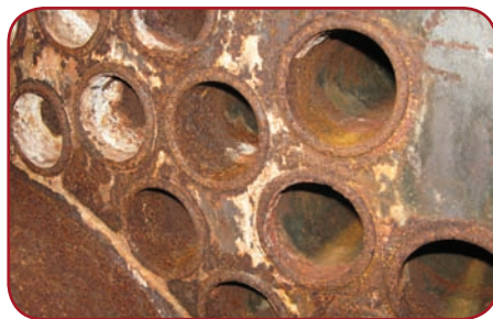
Figure 2. The tubesheet of a boiler that has been in service.
