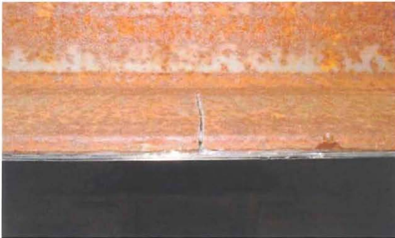
Tension flange cut on both sides of web
