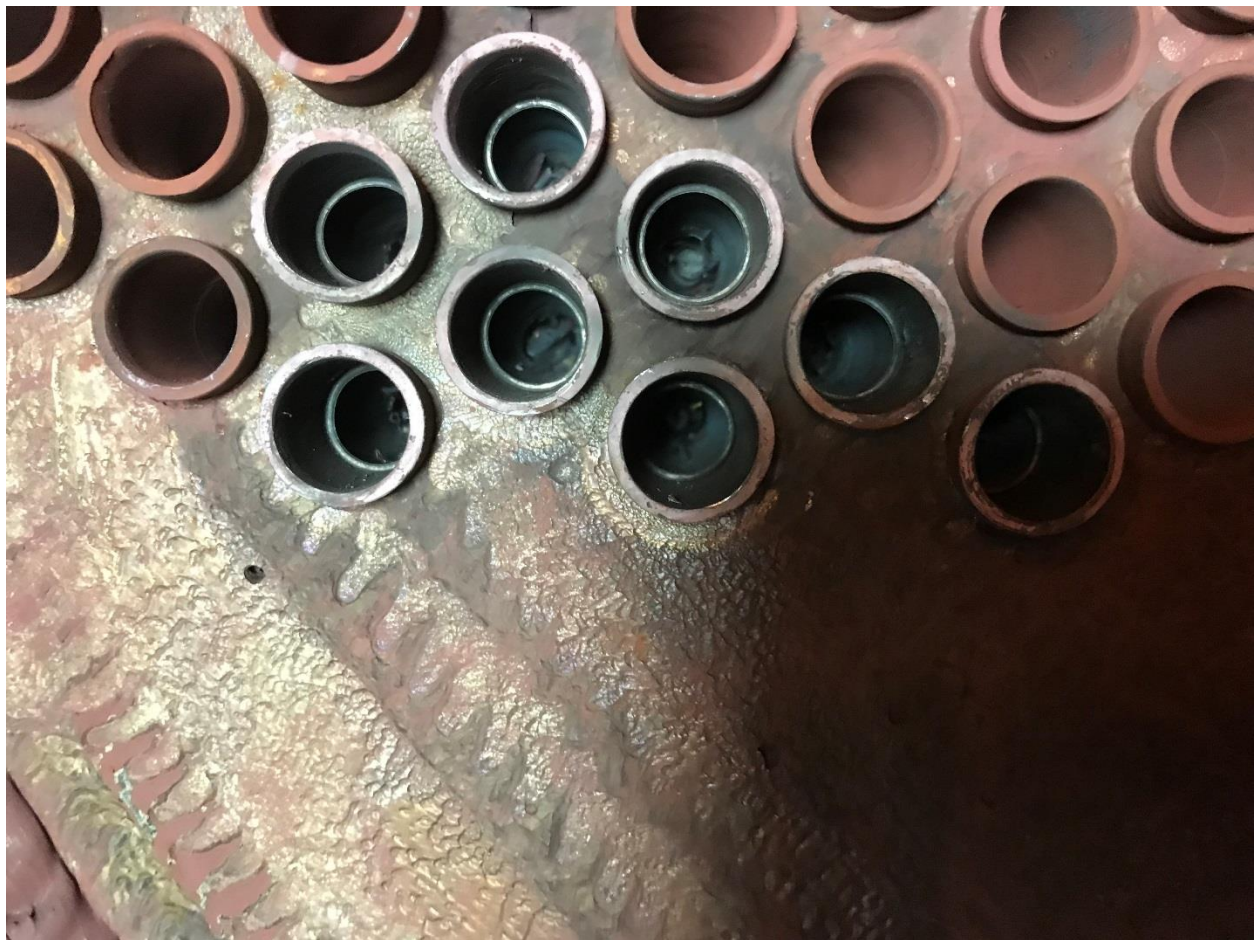
Figure 1 8 Installed Explosive Plugs
