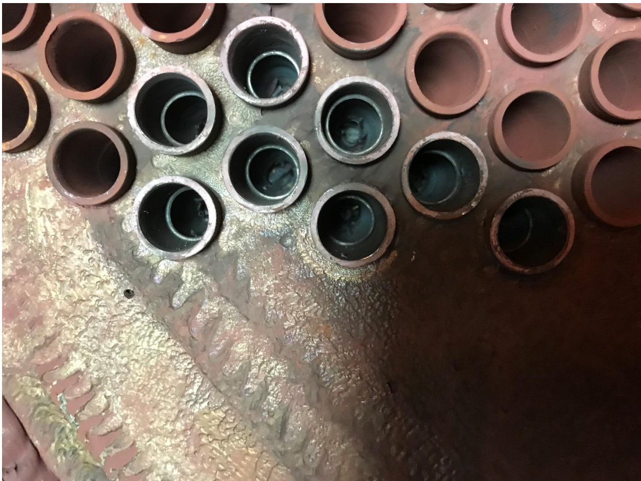
Figure 1 8 Installed Explosive Plugs
