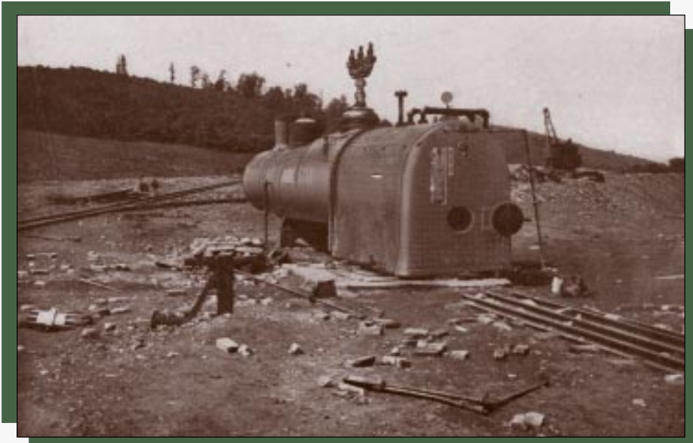
◆ View showing the radial-stay boiler after its low-water test and the distribution of debris over a radius of 175 feet.
