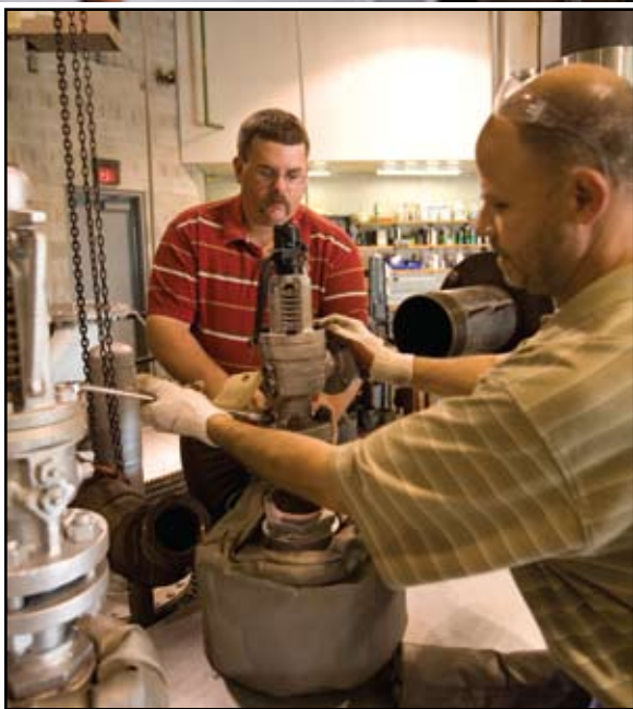
Above, Brandon Ashbrook (left) and Tim Brown hook up a steam pressure relief valve for testing.
