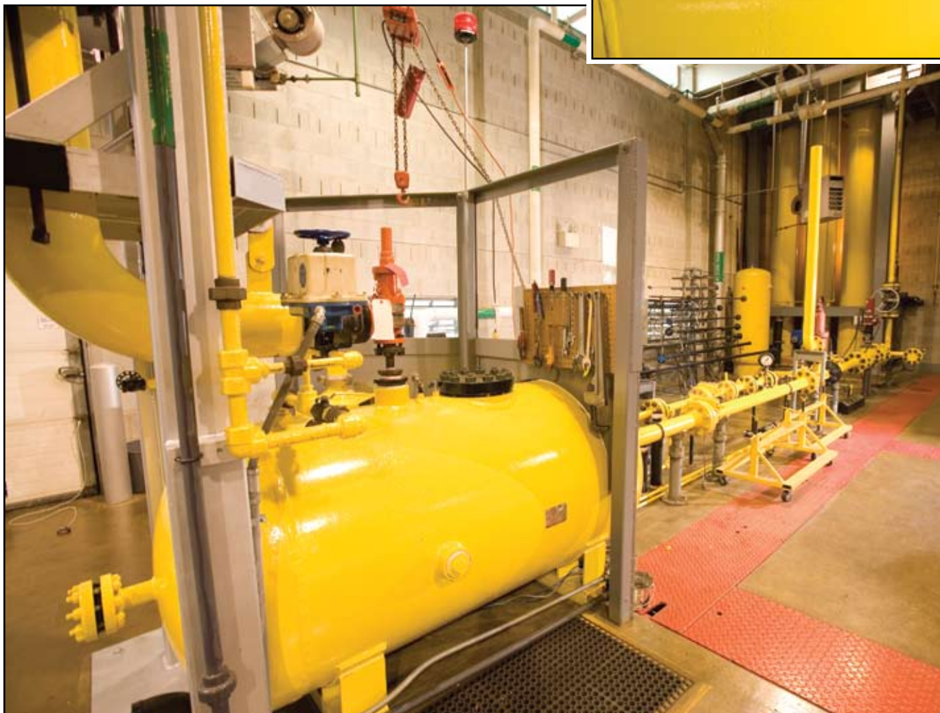
Brandon Ashbrook, right, tests an air pressure relief valve. Shown below, the air pressure test line.
