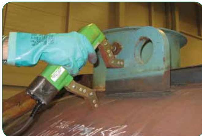
MT examination of a lifting lug weld on an inservice boiler.
