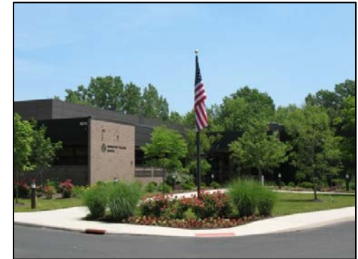
Inspection Training Center
