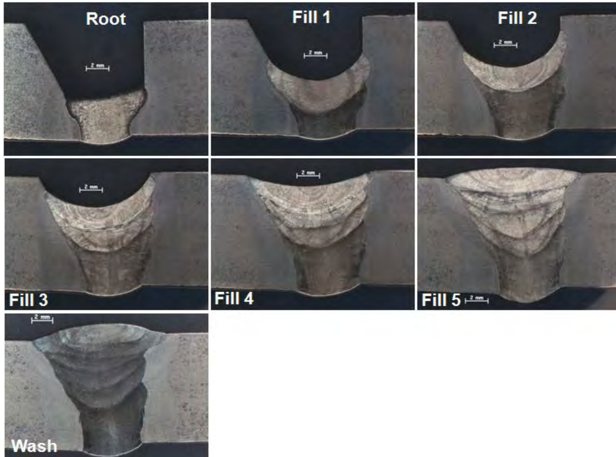
Figure 12 Consistent Layer Weld Passes
