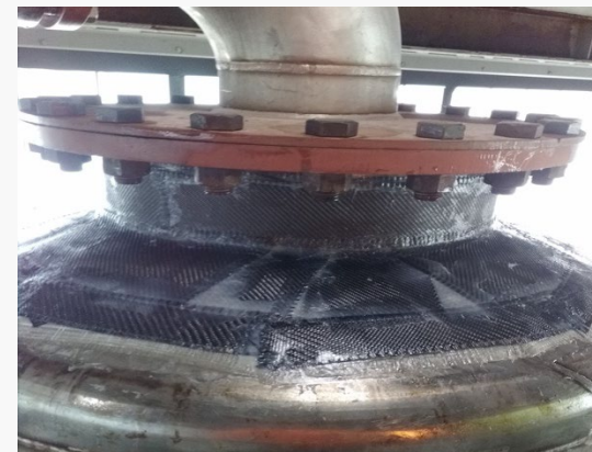
Apply Saturated Carbon Fabric
