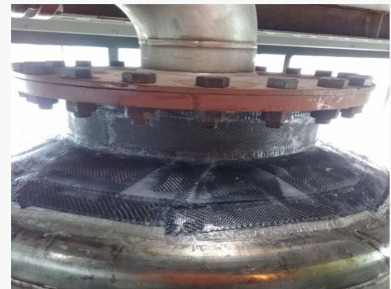
Apply Saturated Carbon Fabric
